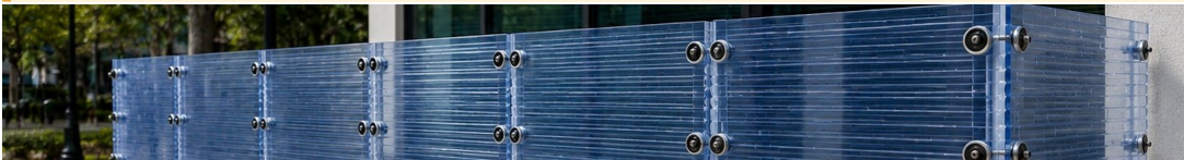
PERIMETER INSTALLATION ON STRUCTURAL FIBERGLASS SUPPORT POSTS
