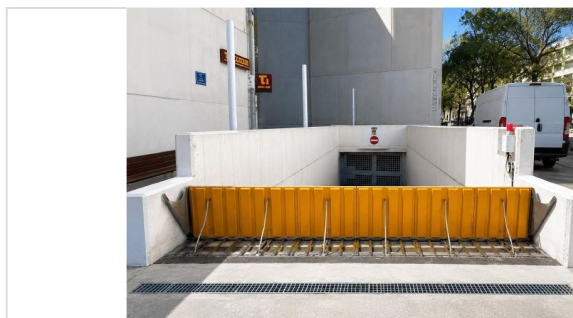
BELOW-GRADE PARKING RAMP — DEPLOYED
