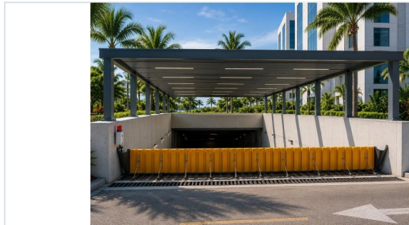
PARKING GARAGE ENTRANCE
