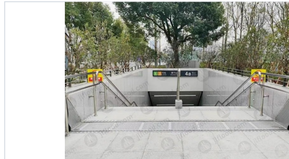
TRANSIT / METRO ENTRANCE
