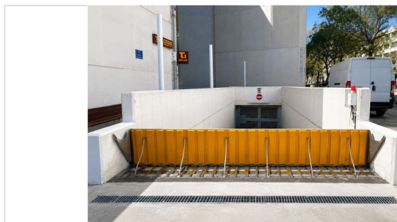
BELOW-GRADE PARKING RAMP — DEPLOYED
