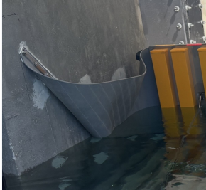
EPDM/silicone side seal flexing against the wall as the panel rises.
