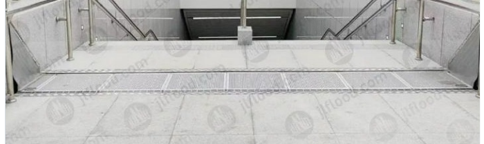
Recessed channel & drain grate, embedded install
