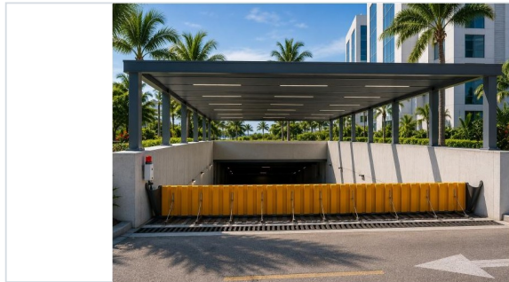
PARKING GARAGE ENTRANCE
